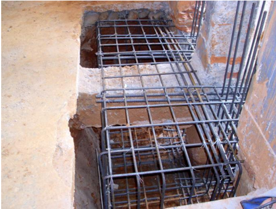
(b) Rebar assembly
