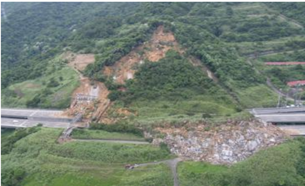
Figure 6.2. National Freeway No. 3 3.1K landslide (Taiwan Geotechnical Society, 2011).
