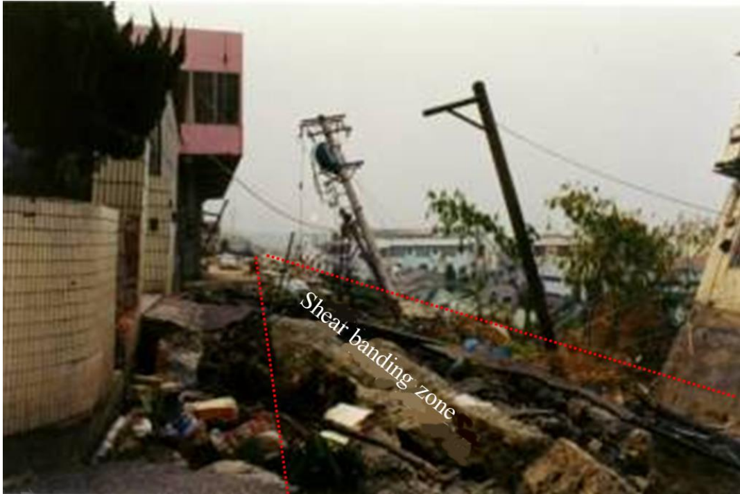
Figure 4.54. Leaning failure of buildings induced by shear banding in 921 Earthquake
