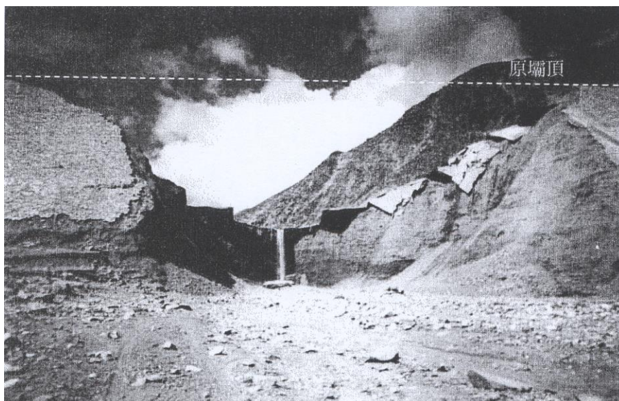
Figure 3.7 Gouhou Dam after dam break (Sinotech Foundation for Research and Development of Engineering Sciences and Technologies, 2008)
