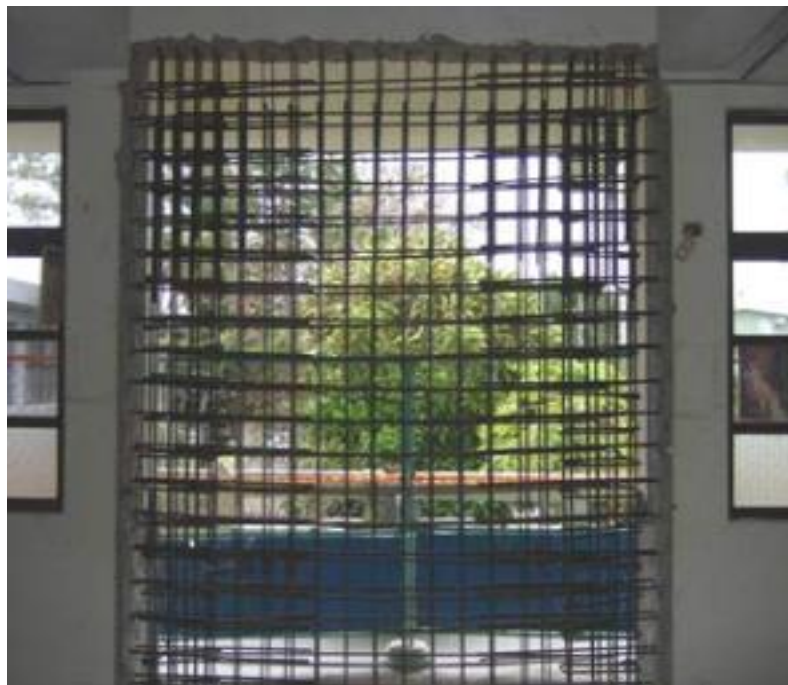
(a) Rebar assembly
