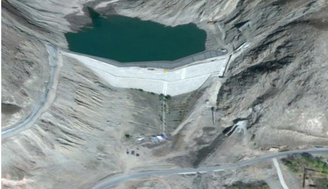
Figure 3.10 Water leakage in the downstream of Gouhou Dam (Google Earth, 2017)
