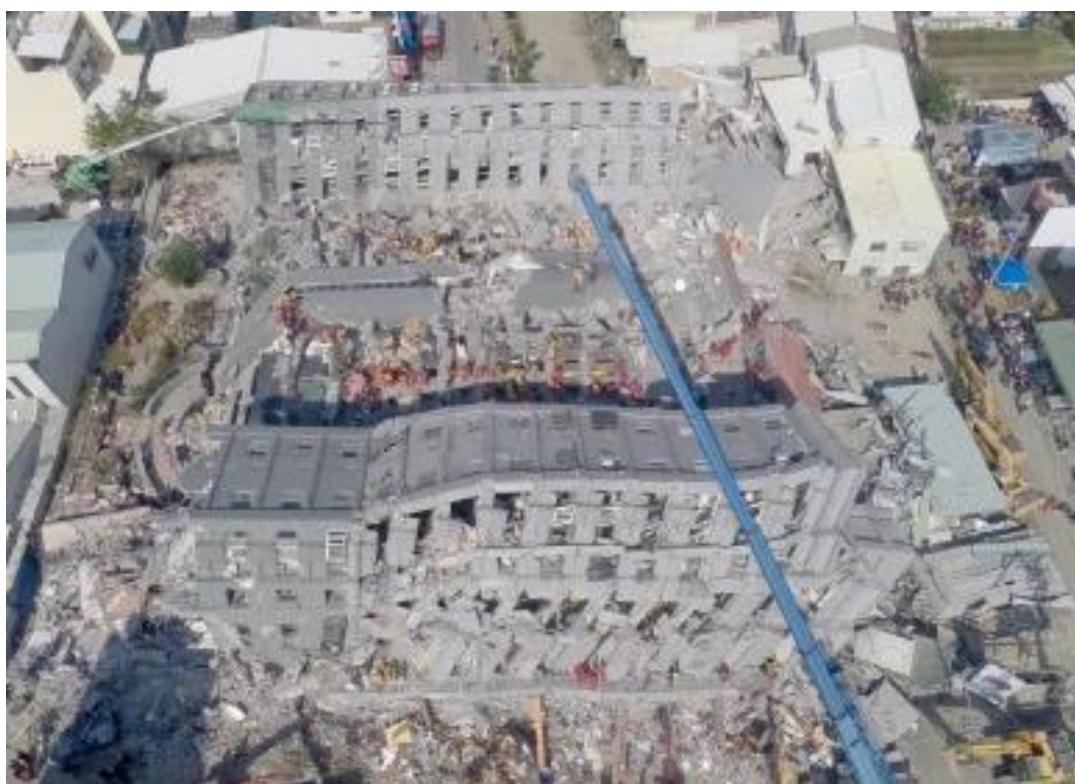
Figure 2.42 Weiguan building after the collapse (Liberty Times Net, 2016)
