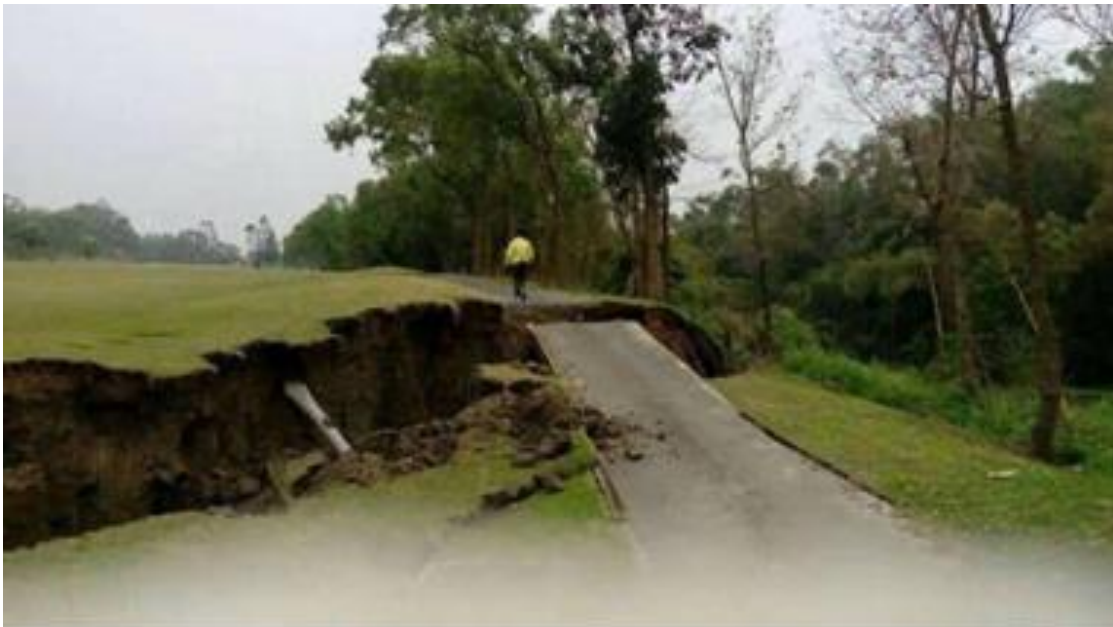
Figure 8.7. Striped soil liquefaction took place during Meinong Earthquake (Liberty Time Net, 2016)
