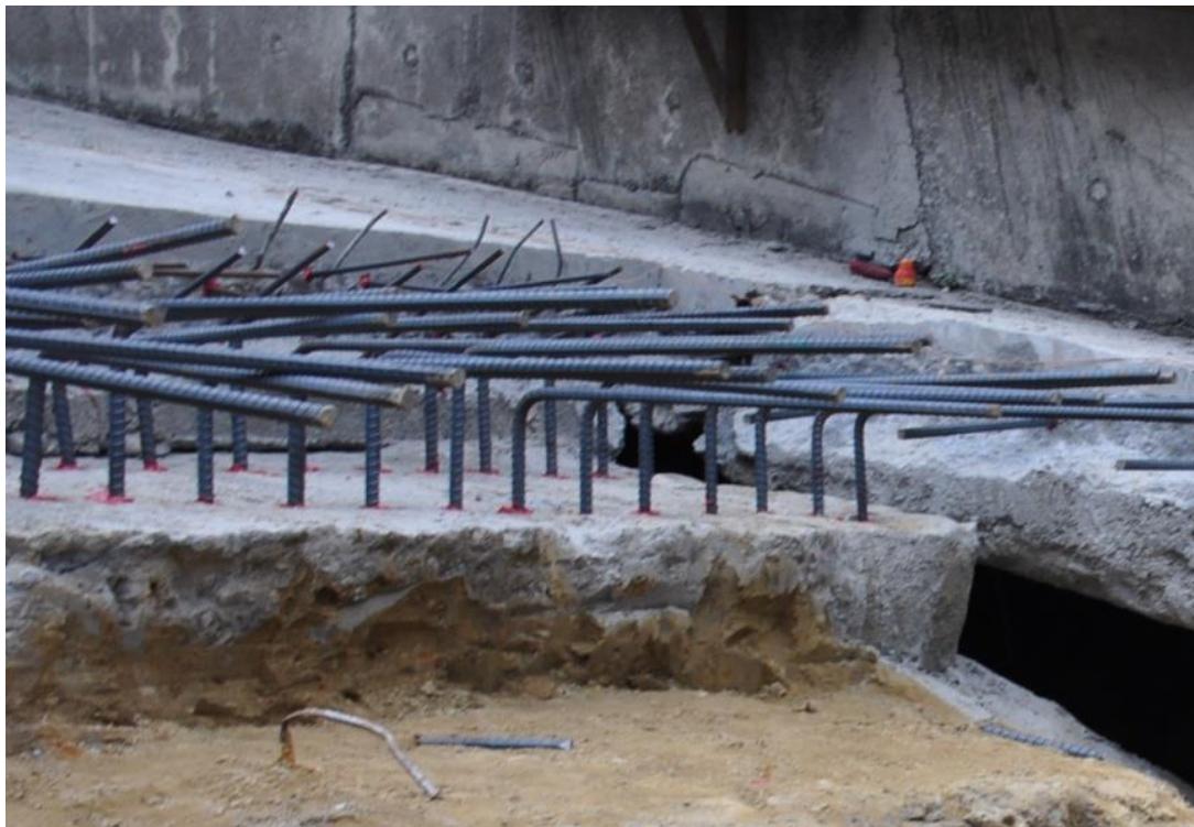
(b) Anti-slip steel bars were added into the repair project
