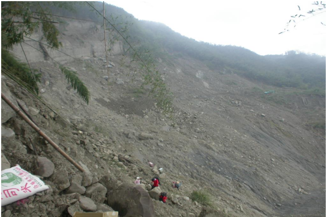
(a) After sliding failure
