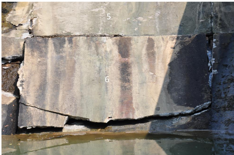
Figure 3.47. The 6th bottom plate and adjacent bottom plates of the spillway
