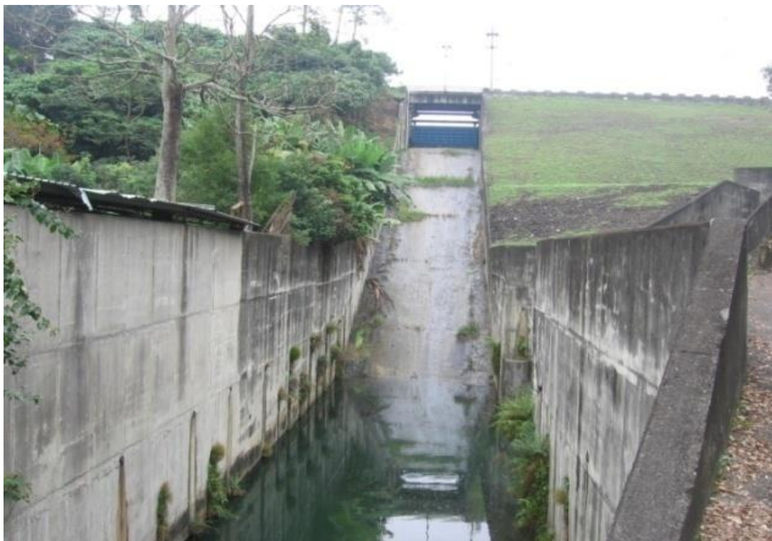
Figure 3.3 Local image of Renyitan Reservoir spillway
