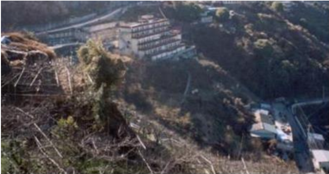
Figure 5.9. Landslide of wedge type on the location of Guest Hotel
