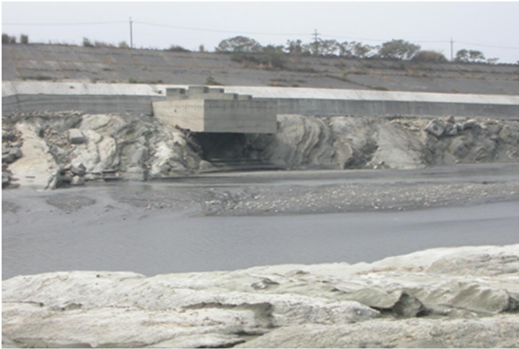
Figure 4.57. Wash-out phenomenon of a shear banding river bank
