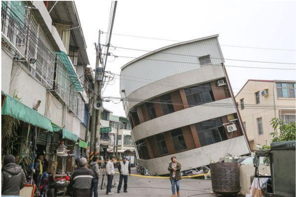
(a) Local tilting of a civil house (New Tang Dynasty, 2016)
