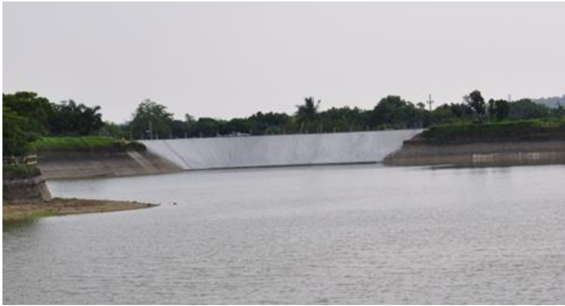
(a) Dam body after emergency repair
