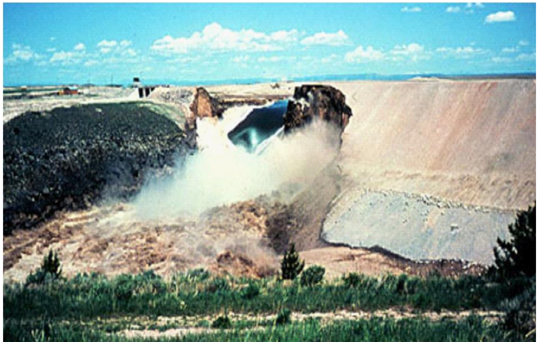
(b) Dam body soils were carried away by the torrent
