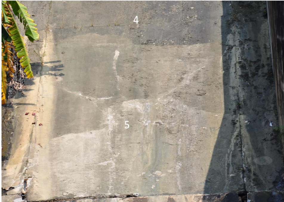
Figure 3.46. The 5th bottom plate and adjacent bottom plates of the spillway
