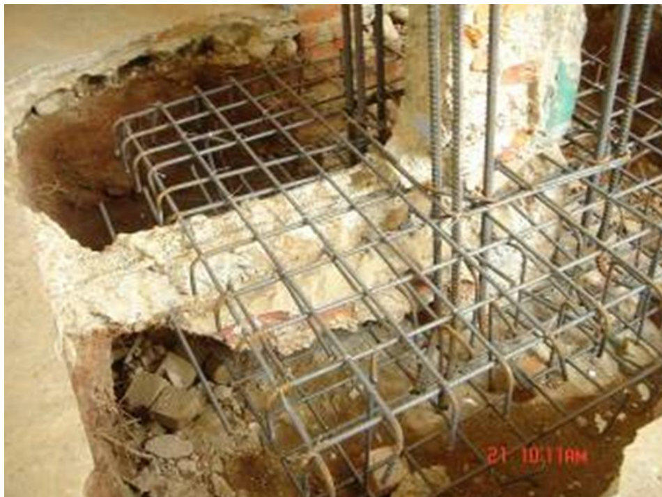
Figure 2.25. Second method of column foundation reinforcement (Chen, 2015)
