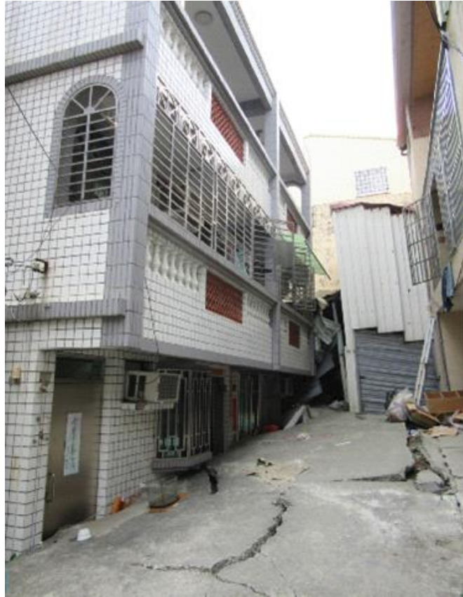
(a) The case of misidentifying the punching shear failure of foundation as soil liquefaction (Lee, Der-Ho, 2016)
