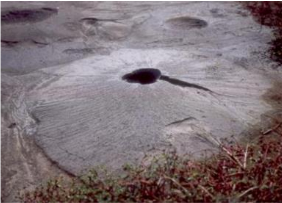
Figure 8.6. Tubular soil liquefaction took place during Chi Chi Earthquake (EOU Education Market, 2014)
