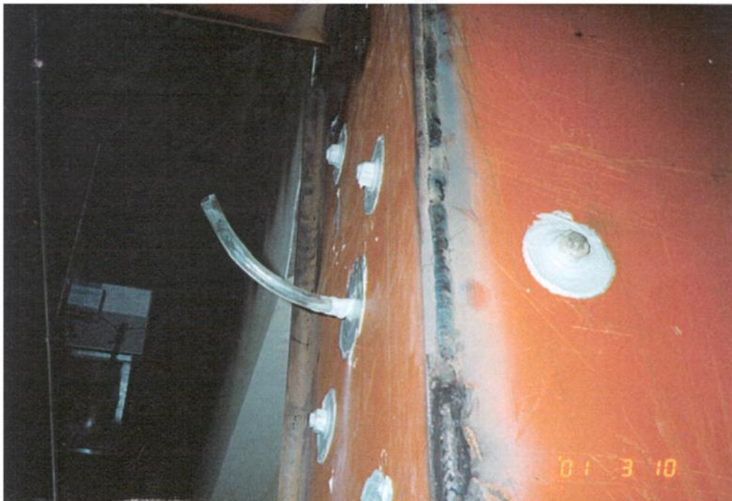
(b) Wrapping with steel sheet
