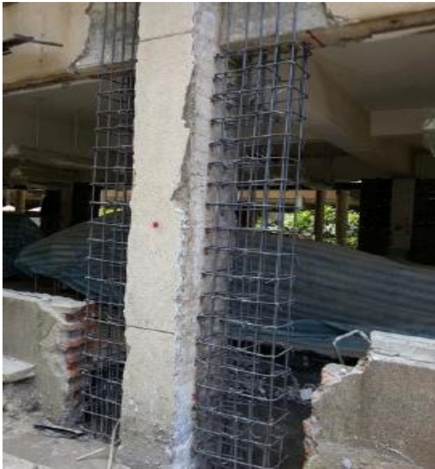
(a) Rebar assembly (Ting-Wei Hsu, 2011)
