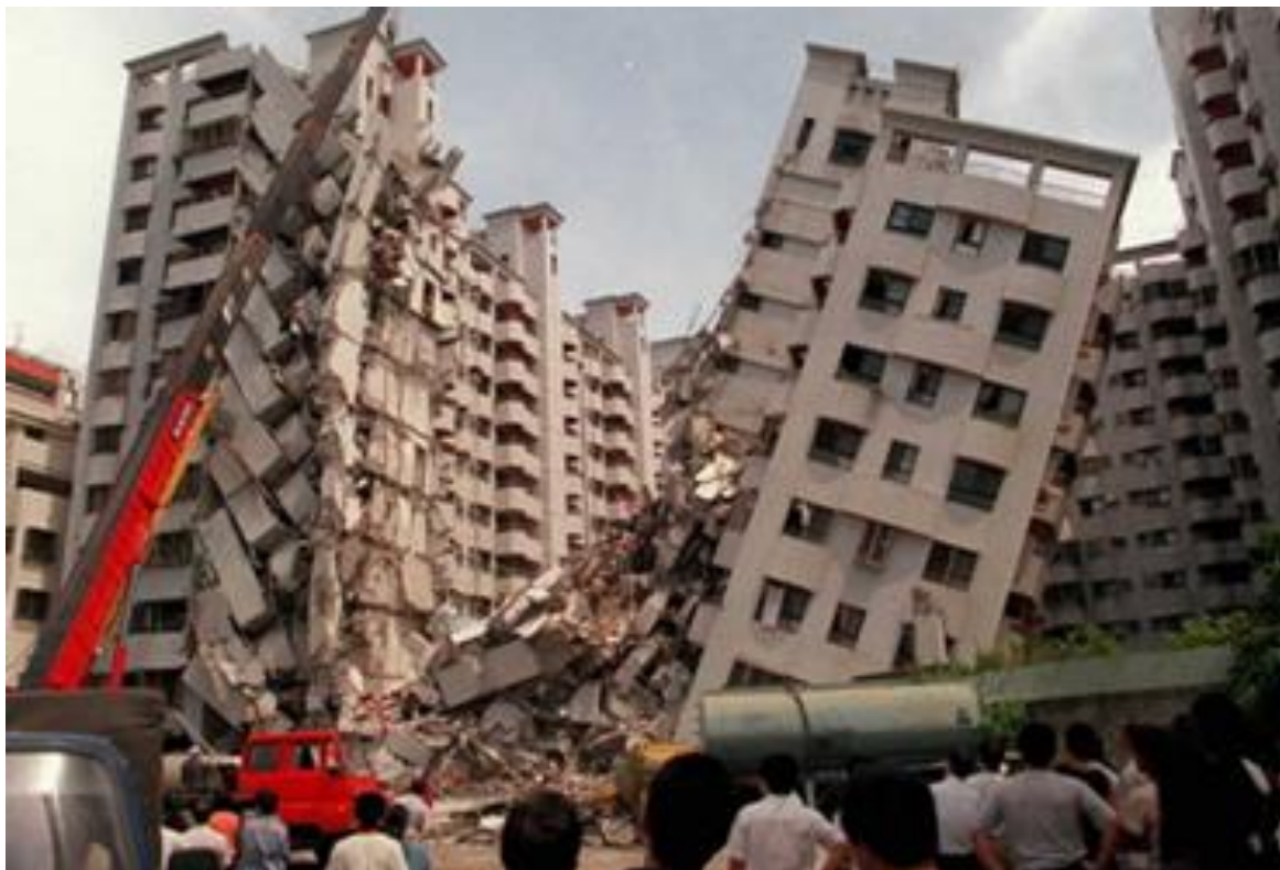
(b) Actual building damage pattern (Pixnet, 2010)
